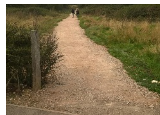
Improvements to the surface of footpath 11 from School Green to Deardon Way, achieved by the Shinfield Volunteer Group, in collaboration with the Parish Council and Buxted Construction
