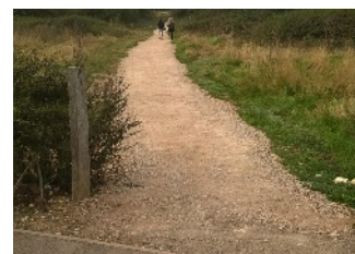
Improvements to the surface of footpath 11 from School Green to Deardon Way, achieved by the Shinfield Volunteer Group, in collaboration with the Parish Council and Buxted Construction
