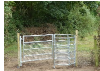
A new kissing gate funded by the Parish Council and installed by the Loddon Valley Ramblers group at Langley Mead SANG to provide a mud-free entrance into the SANG from Millworth Lane
