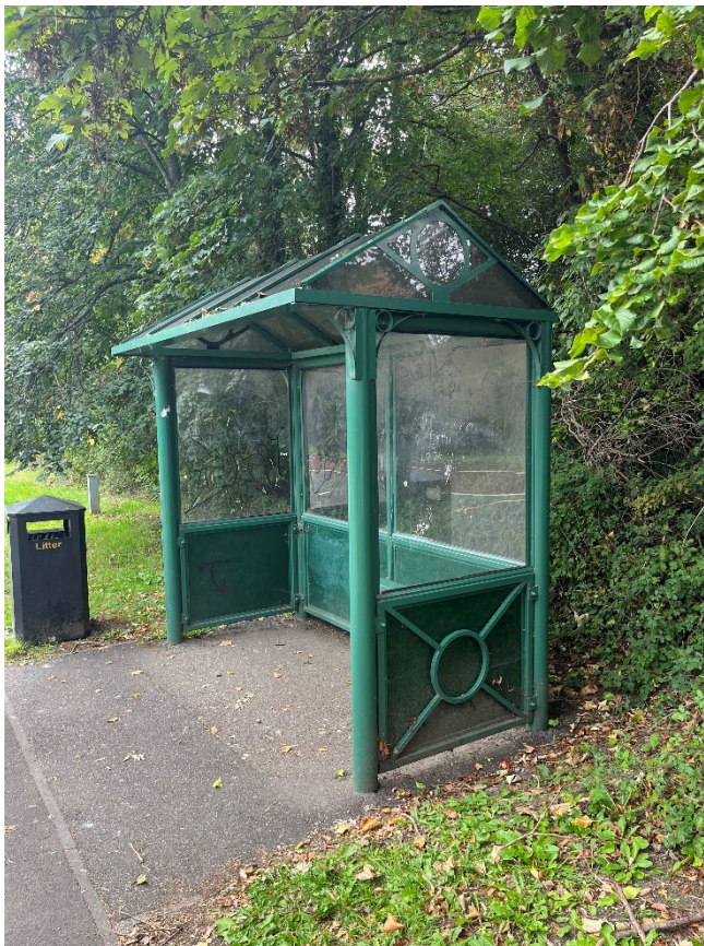
This style is on Hollow Lane, opposite side of the one that needs replacing.
