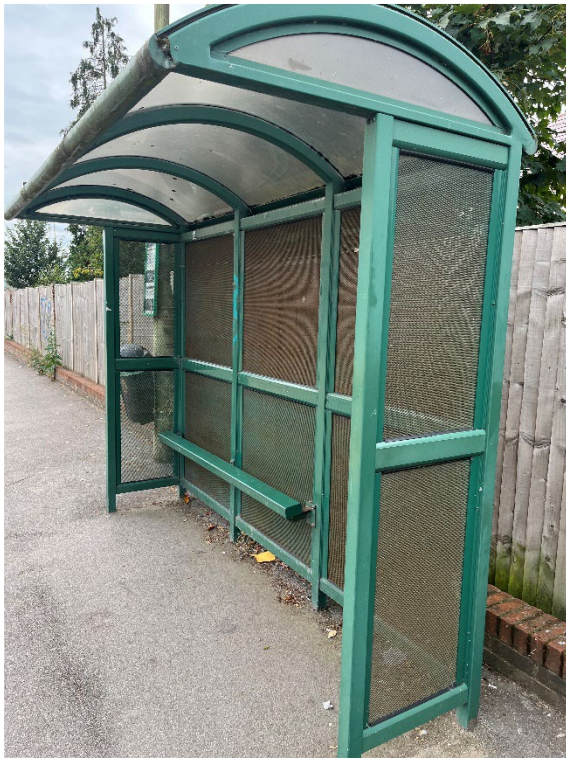
Example of bus shelter on Shinfield road with anti-graffiti polycarbonate panels
