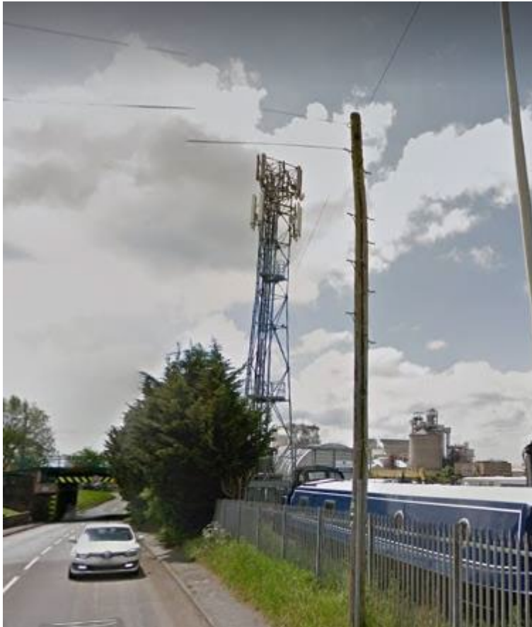
Figure 2 Example of a shared lattice tower next to the road.
