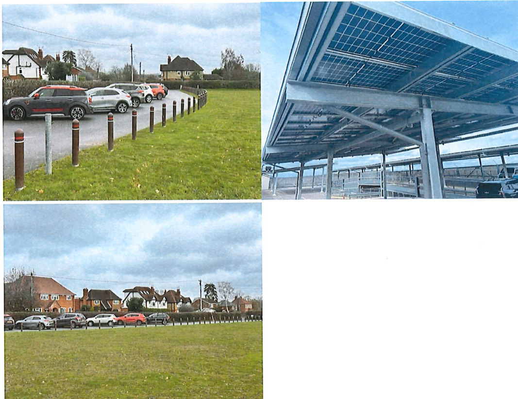
Spencers Wood Pavillion Parking & a typical solar canopy construction
