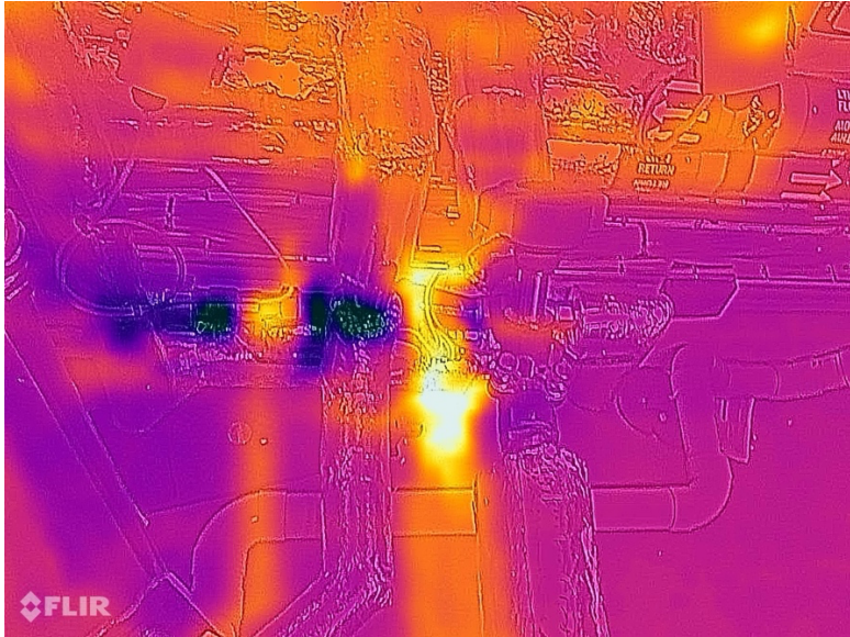
Missing valve insulation in plant room, refit.
