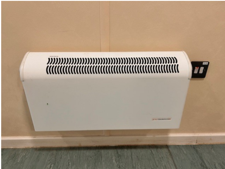
Consort heater – programmer required / re-set
