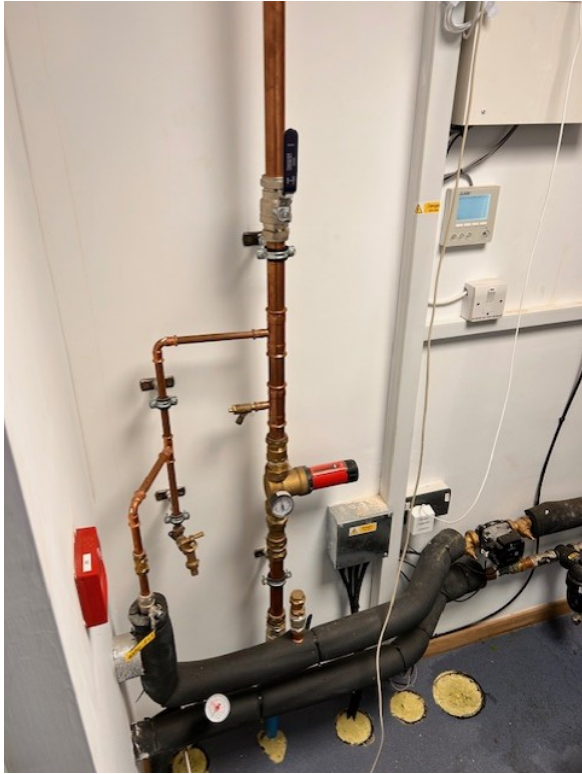
Uninsulated pipework
